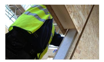
Racking resistance of a SIP wall is typically 50% greater than that of a timber studwork wall sheathed with one layer of 9mm OSB. Therefore a low rise building designed to be constructed with loadbearing timber studwork, should also work as a loadbearing SIP structure. A structural engineer would need to confirm this by calculation.
